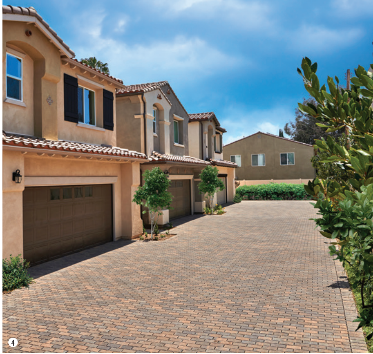
1. Permeable Holland in Gray-Moss-Charcoal installed in a running bond pattern. 2. Permeable Holland in Sand (special order color) installed in a running bond pattern. 3. Gray-Moss-Charcoal Permeable Holland machine laid in a herringbone pattern. 4. Permeable Holland in Tuscan (special order) installed in a running bond pattern. Border is Permeable Holland in Tuscan installed in a soldier course.
