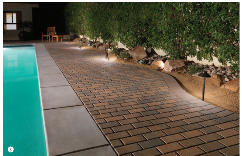
1. Holland in Gray-Charcoal installed in a 45 degree herringbone pattern. Note: This stone was manufactured at 80mm due to site conditions and anticipated traffic loads. 2. Gray-Charcoal Holland installed in a herringbone pattern. 3. Cream-Brown-Charcoal Holland installed in a running bond pattern with a solid Mocha Holland border at the landscape edge. 4. Gray-Charcoal Holland installed in a running bond pattern. Border is Holland Gray-Charcoal in a soldier course.
